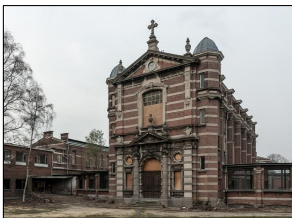
Rys. 132. Kaplica szpitalna na terenie Militair Hospitaal, Antwerpia, 2007. Fig. 132. Hospital chapel on the area of the Militair Hospital, Antwerp, 2007.
